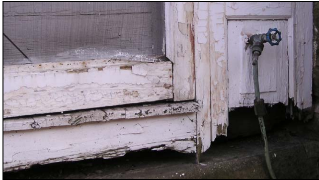
The wood base is in contact with the concrete foundation. Regular wood dampness can eventually lead to rot and deterioration.
