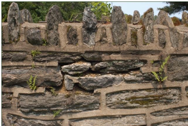
Stone walls are an important historic feature in the Village of Roslyn. Large areas of missing mortar allow water to penetrate the wall and support plant growth. The moisture infiltration and plant roots can further deteriorate the wall by popping-out pointing mortar.
