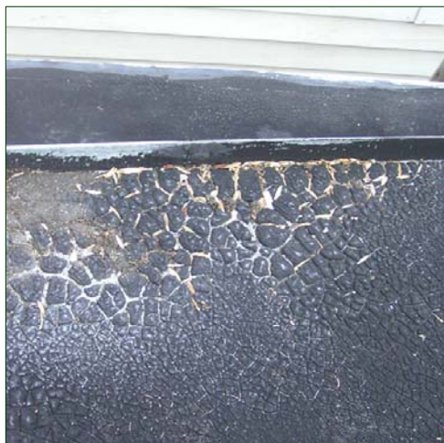
The alligatored roof surface indicates roof deterioration and possible need for replacement.
