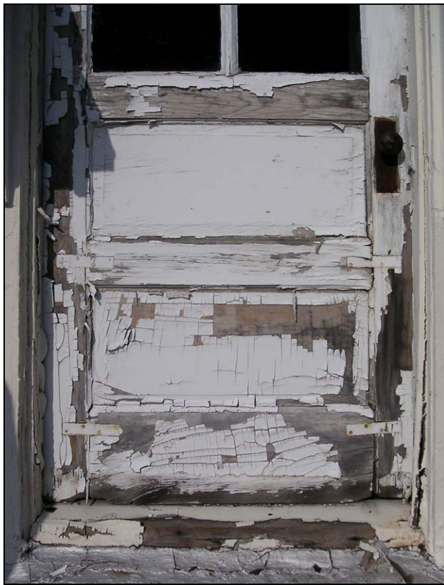
The paint on this door has alligatored, and severe cracking is visible. Removal of paint down to bare wood and proper door repair are recommended prior to repainting
