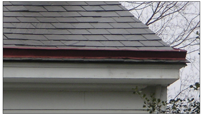
Pole gutters, also known as parallel gutters or “Yankee” gutters, are built-in gutters located near the roof edge to capture rain water and direct it towards a downspout. They are typically formed of wood, placed vertically to the slope of the roof and wrapped in metal flashing.
