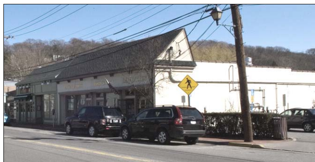
This commercial building has a “decorative” side gable roof at the front elevation, but the majority of the building has a flat roof.
