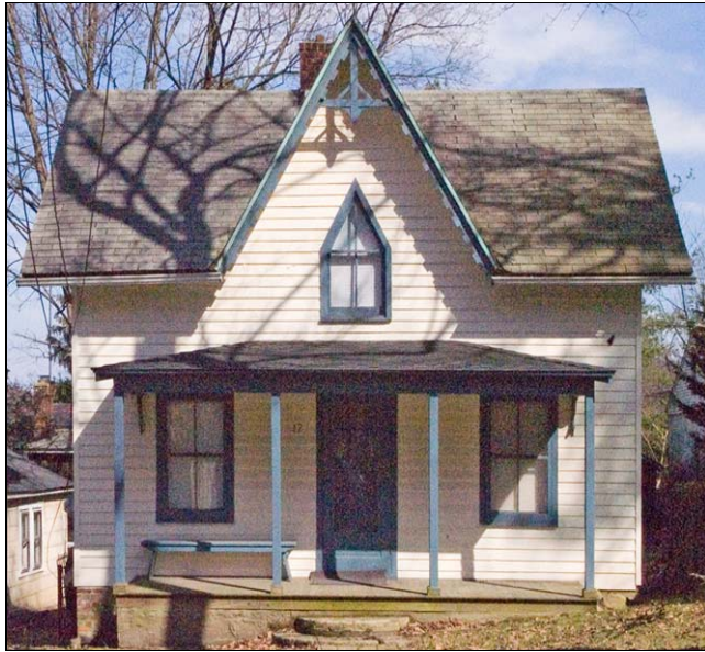
Roof forms, such as this side gable roof with an intersecting front gable, are an important feature in defining a building's style. In this case, the roof forms and detailing of the barge board and gable end, help to identify it as a Gothic Revival cottage. The porch has a shallow half-hipped roof.
