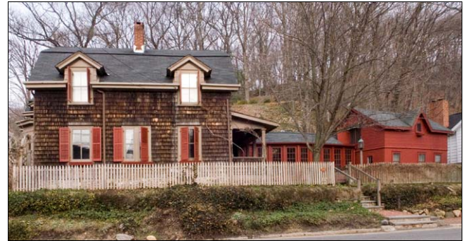
The gambrel roof is a distinguishing stylistic element of this Dutch Colonial Revival house. Various roof shapes are used at the later additions including a shed roof porch, a side gable roof addition with an intersecting gable at the front elevation at the secondary block.
