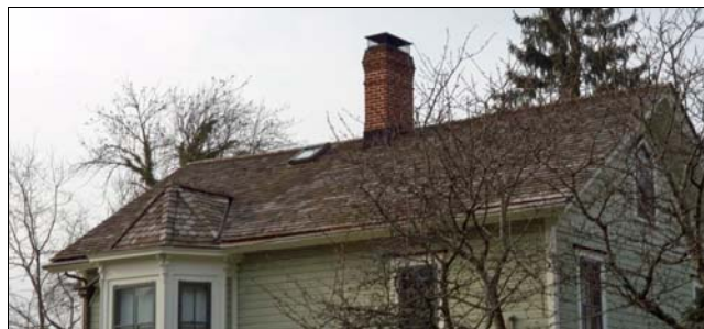
Wood shingles are a locally traditional roofing material.
