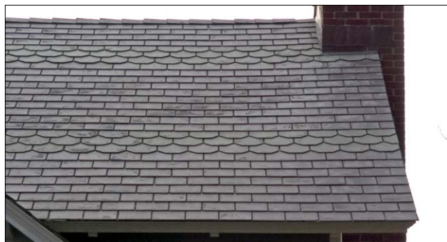
Slates are available in a variety of shapes and colors. The most common color in the Village of Roslyn is grey.
