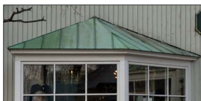
Standing seam metal roofing is a durable material that provides additional texture to this roof.
