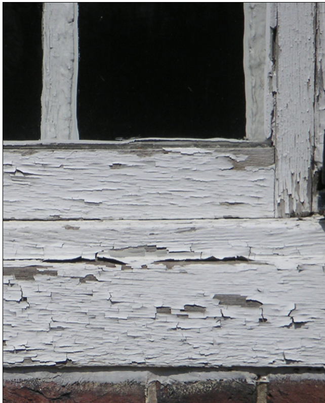
The window sill and jamb have peeling paint and some checking or splitting. Note the open joint between the wood sill and brick.
