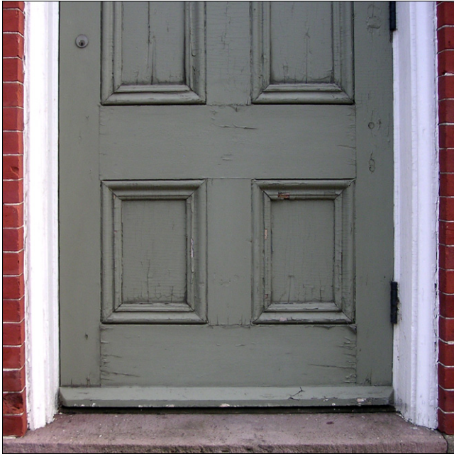
Wood checking and peeling paint visible. Minor repair and maintenance can prolong the serviceable life of this historic door.
